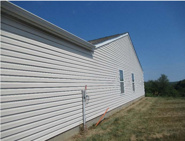
Side elevation and the patio units
