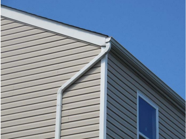
Typical gutter and downspout assembly at Tuscany Estates
